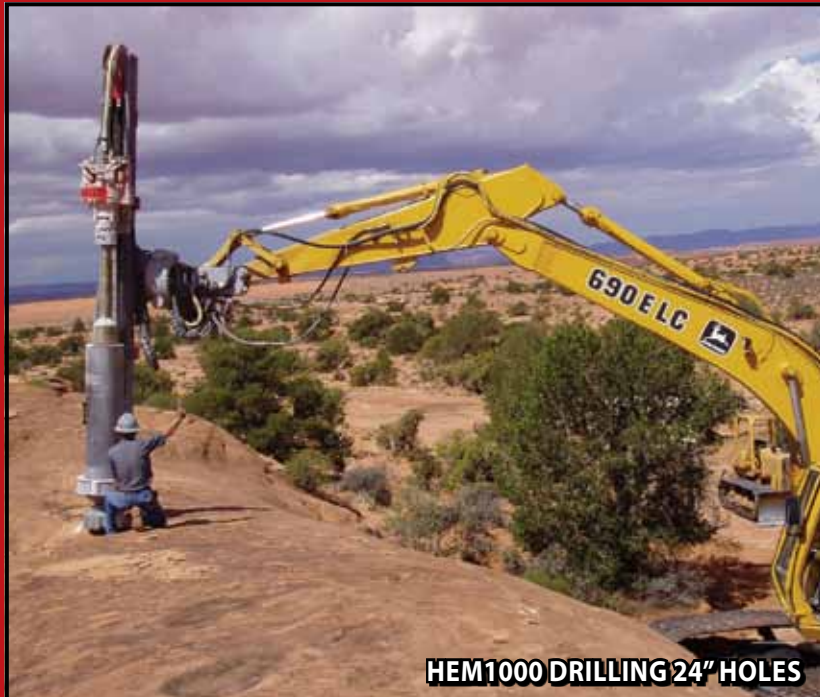
HEM INSTALLING HOLLOW BAR SOIL NAILS
